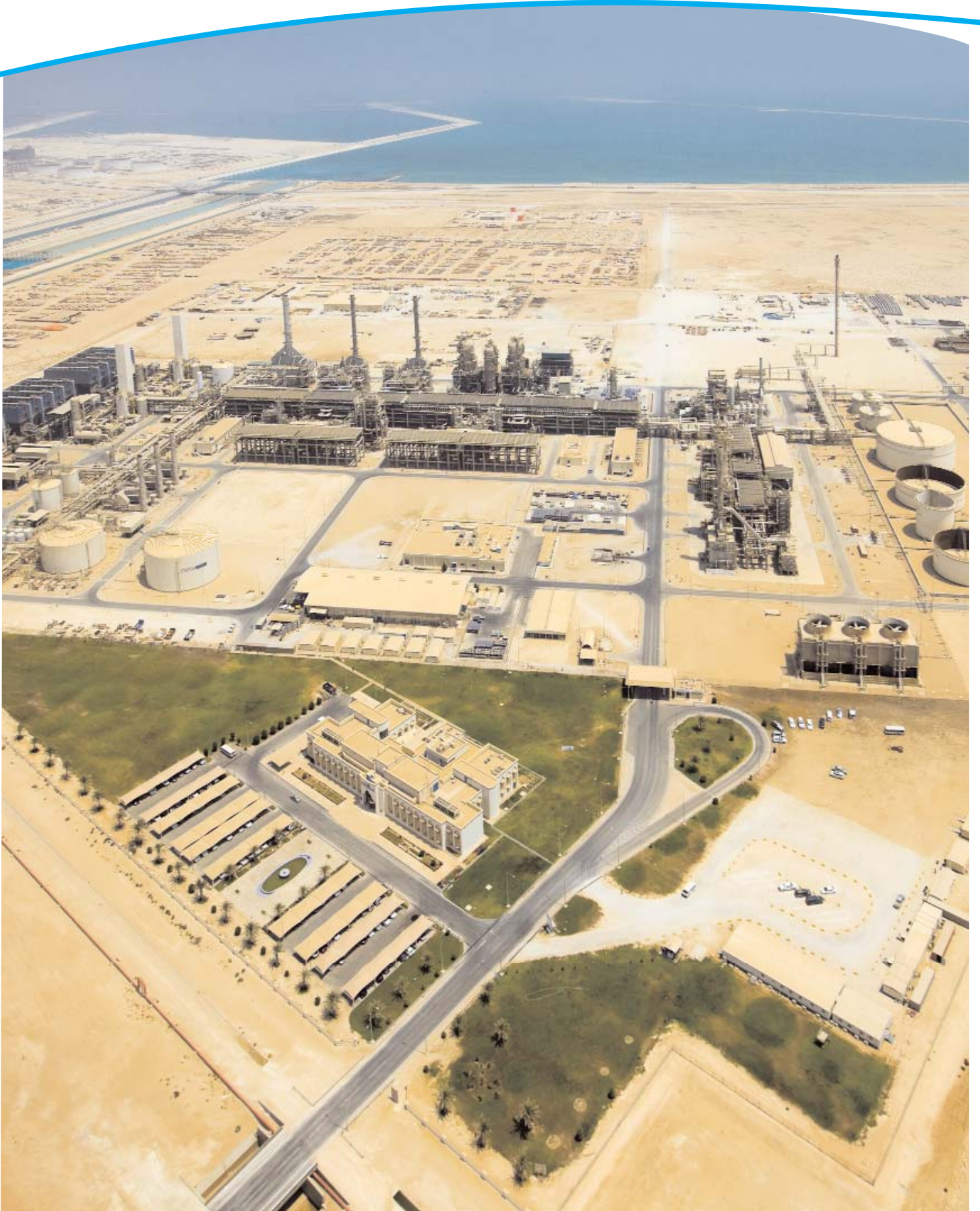
The success of Oryx GTL in Qatar is creating growing interest globally for similar projects.
