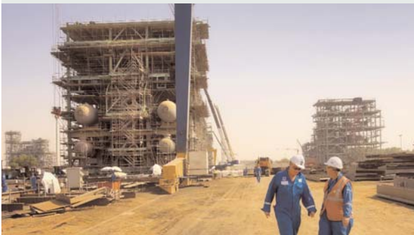
Modular construction of EGTL plant components in Abu Dhabi.
