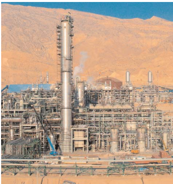
Arya Sasol ethane cracker in Iran begins beneficial operation.
