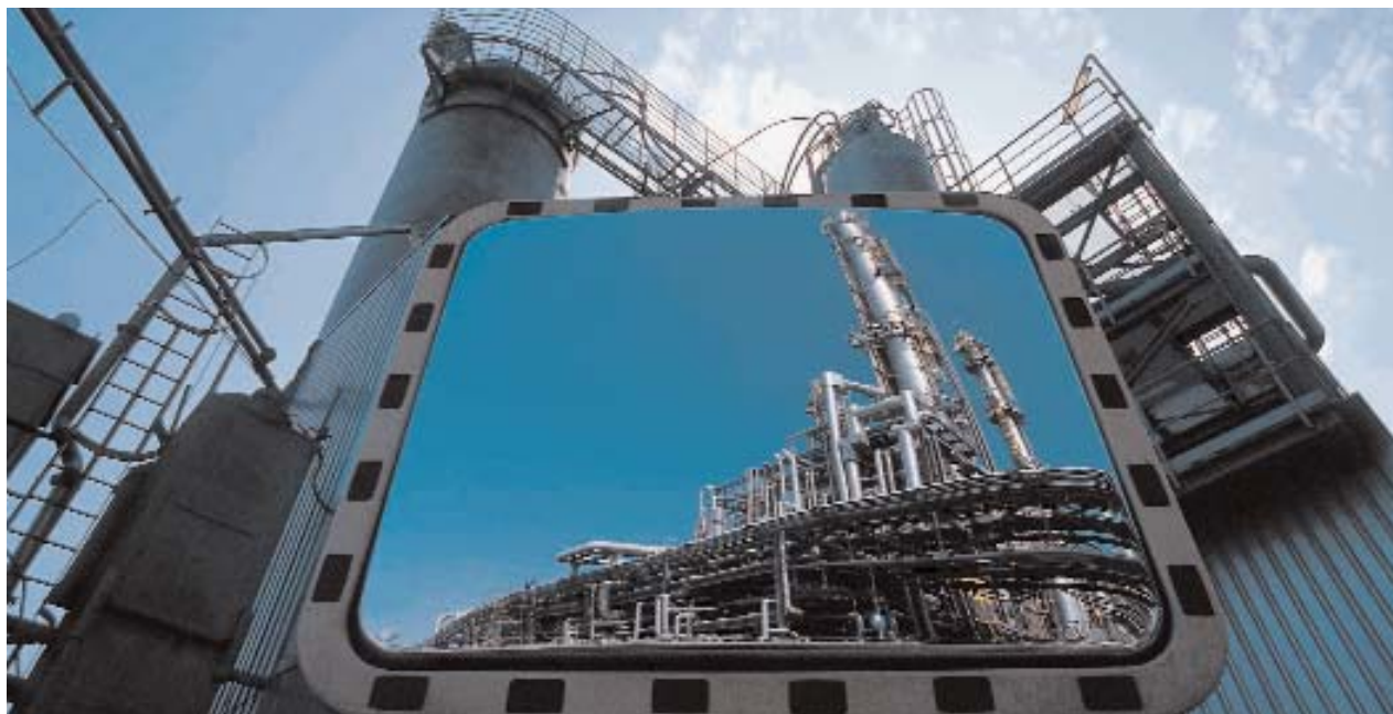
Impressions of the Sasol Olefins & Surfactants site, Brunsbüttel, Germany.
