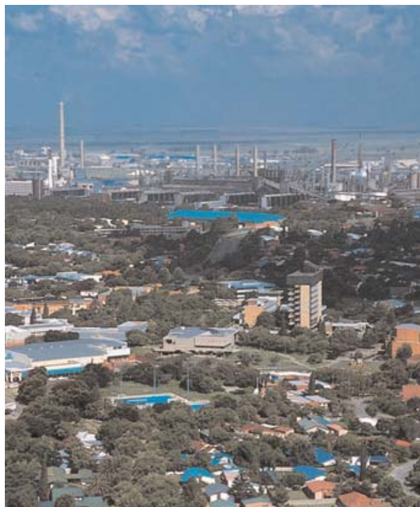
Sasol Infrachem provides feedstock to Sasol’s chemical businesses, as well as utilities and services to operations in Sasolburg.
