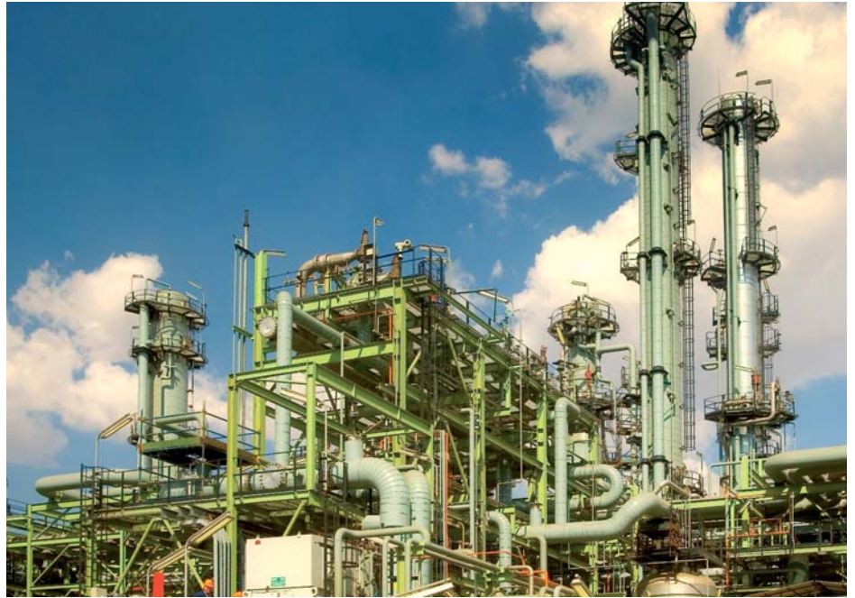
Project Turbo, Sasol's largest capital project in South Africa since its main synthetic fuels plants were built.
