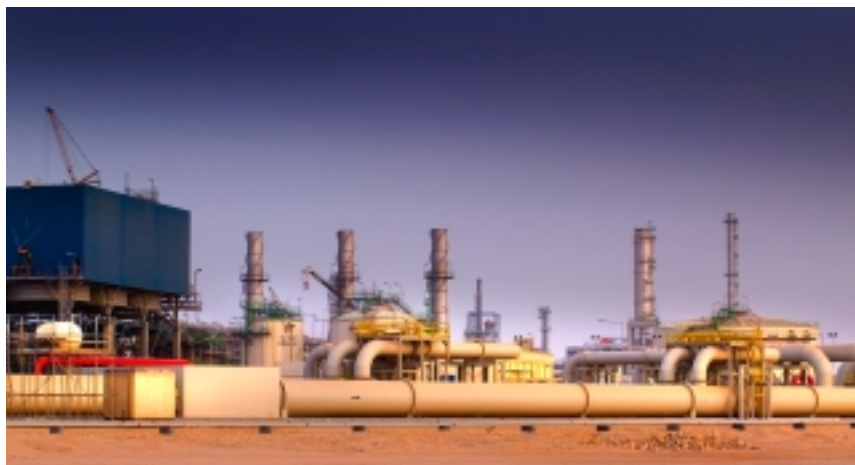
The Oryx GTL plant is nearing completion
