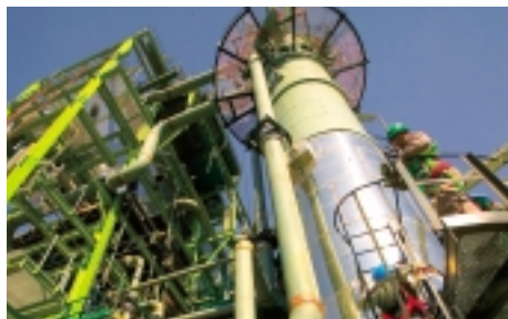
Turbo work in progress
