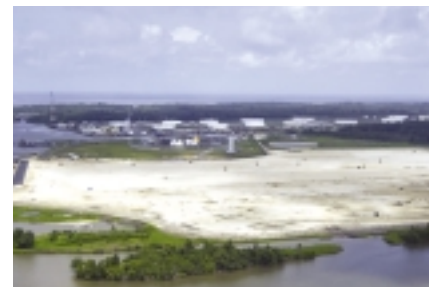
The site prepared for the EGTL plant
