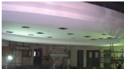
Part of the Oryx GTL facilities being built
