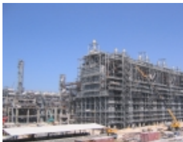
Arya Sasol plants under construction
