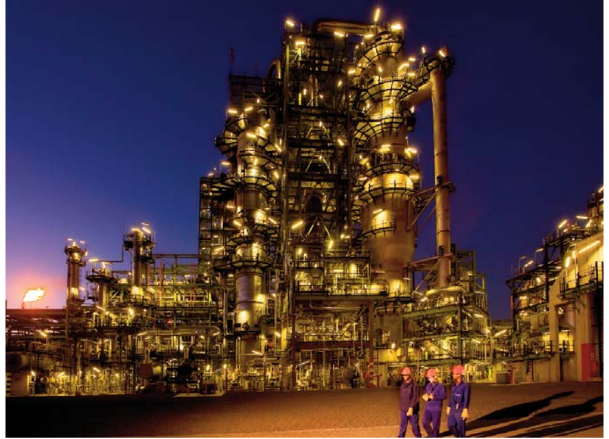
Sasol's selective catalytic cracker portion of project Turbo has produced fit-for-purpose ethylene and propylene
