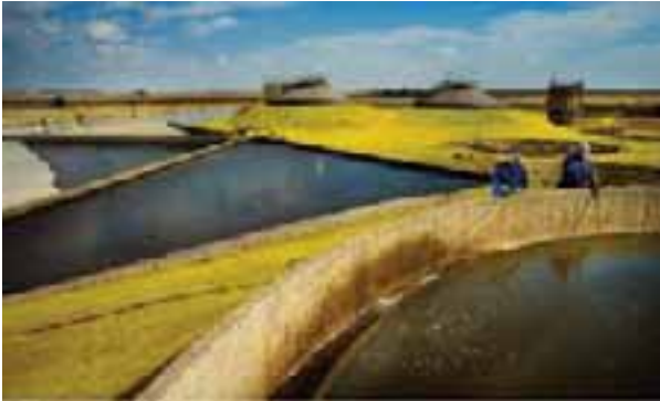
Sasol One water treatment facility
