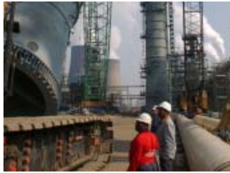
Second Octene train – lifting the tallest distillation column in Africa.
