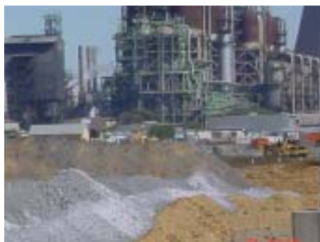
Project Turbo construction site at Secunda.
