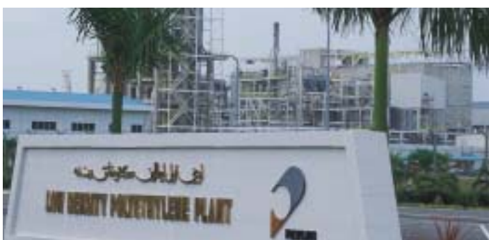
Petlin low-density polyethylene plant at Kertih, Malaysia.
