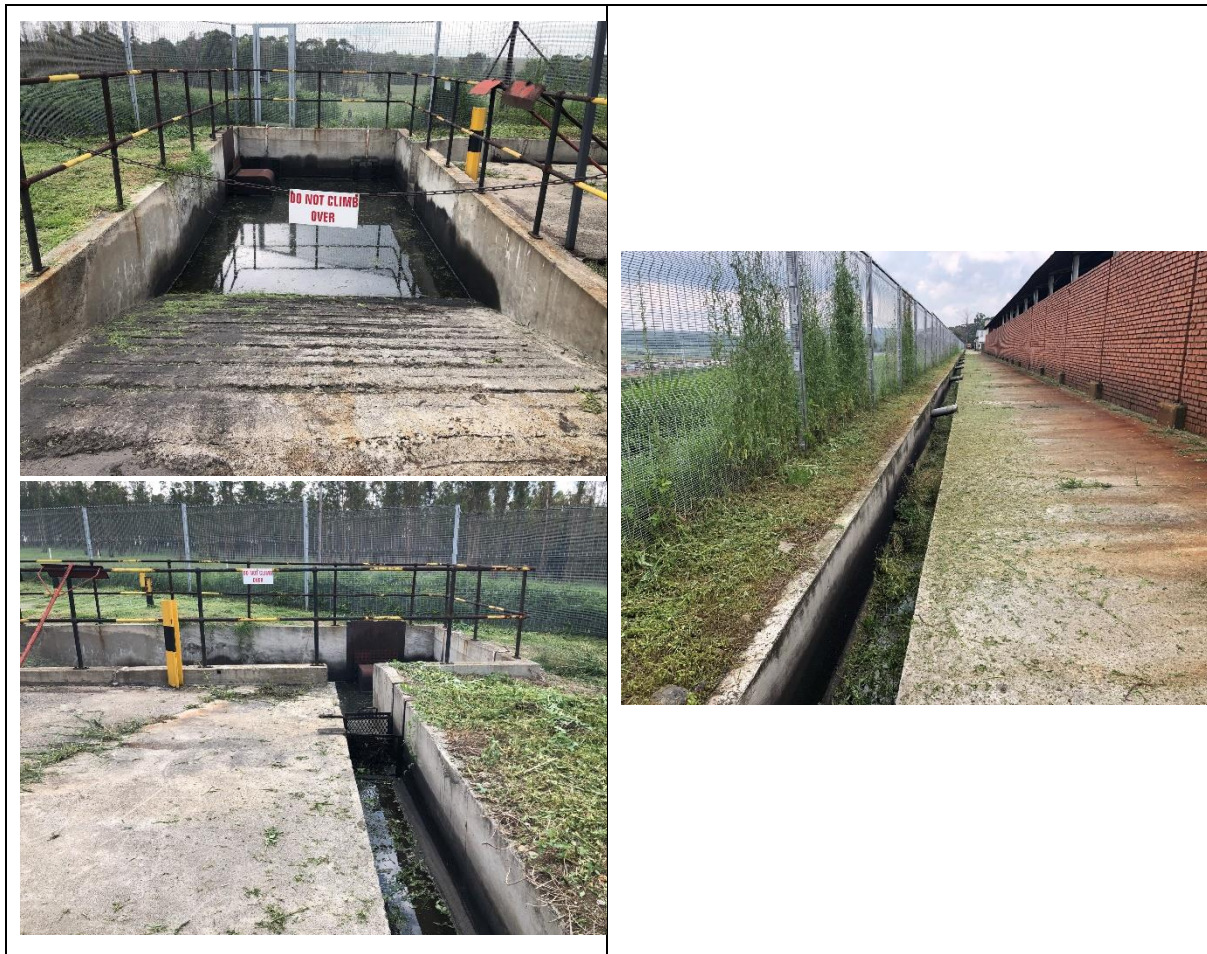
Figure 10-4: Stormwater Trench and Sump at Main Shaft
