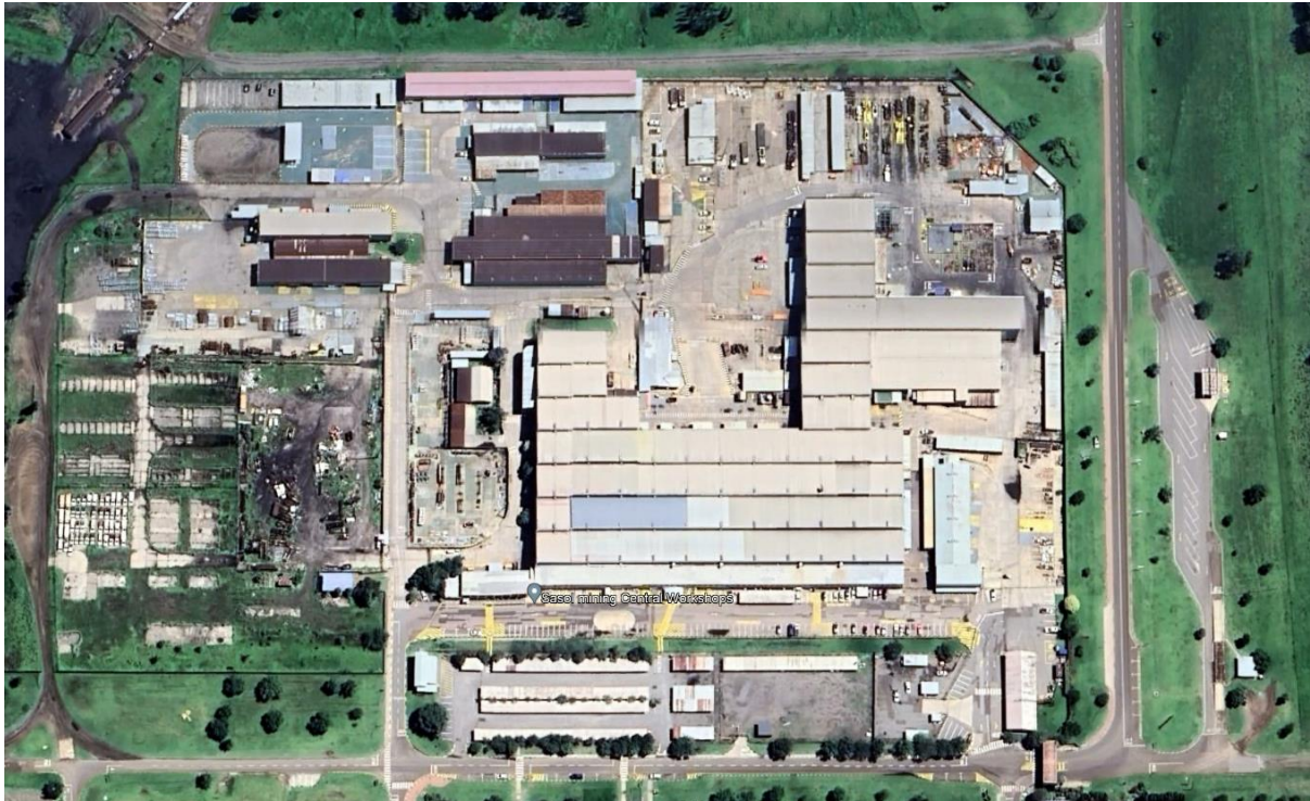
Figure 10-8: Brandspruit Central Workshop
