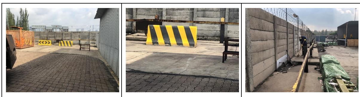
Figure 10-11: Steel Plates Used to Seal the Outflows in the Wall
