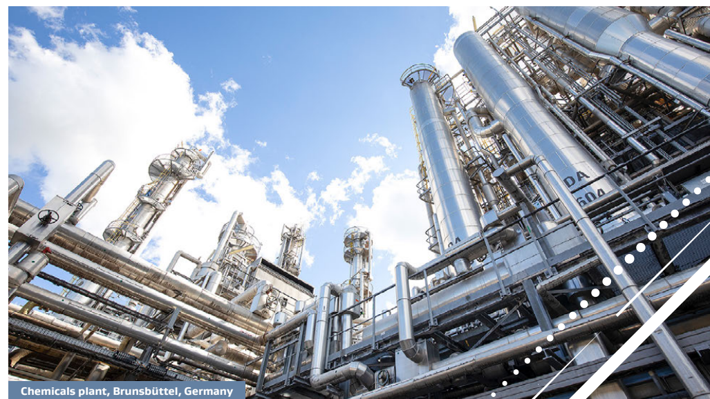
Chemicals plant, Brunsbüttel, Germany
