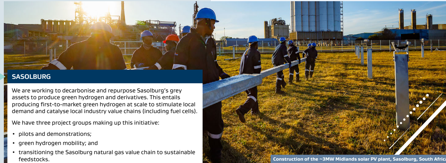
Construction of the ~3MW Midlands solar PV plant, Sasolburg, South Africa
