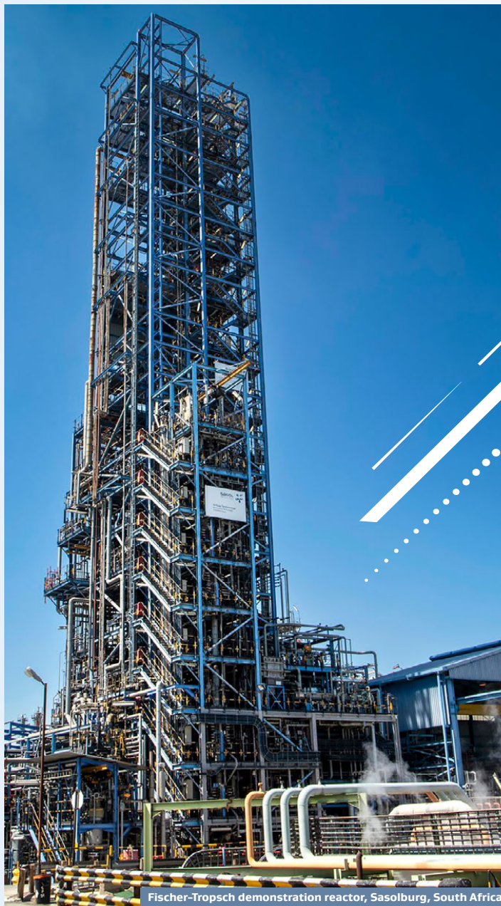
Fischer-Tropsch demonstration reactor, Sasolburg, South Africa
