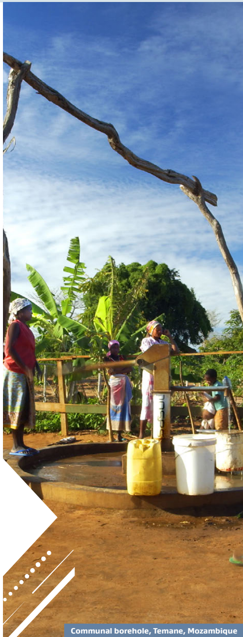
Communal borehole, Temane, Mozambique
